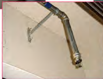
Fire rated spandrel wall
