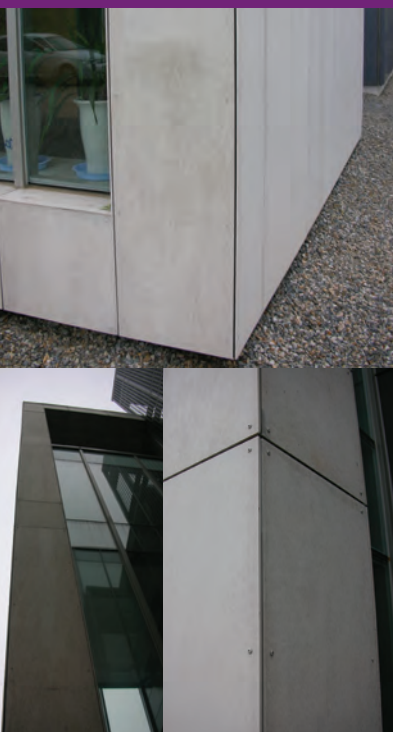
Undecorated building façade
