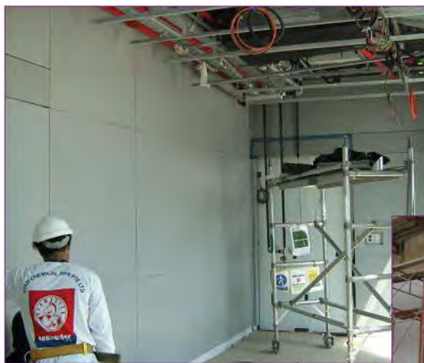
Interior cladding with factory-applied polyurethane paint finish
